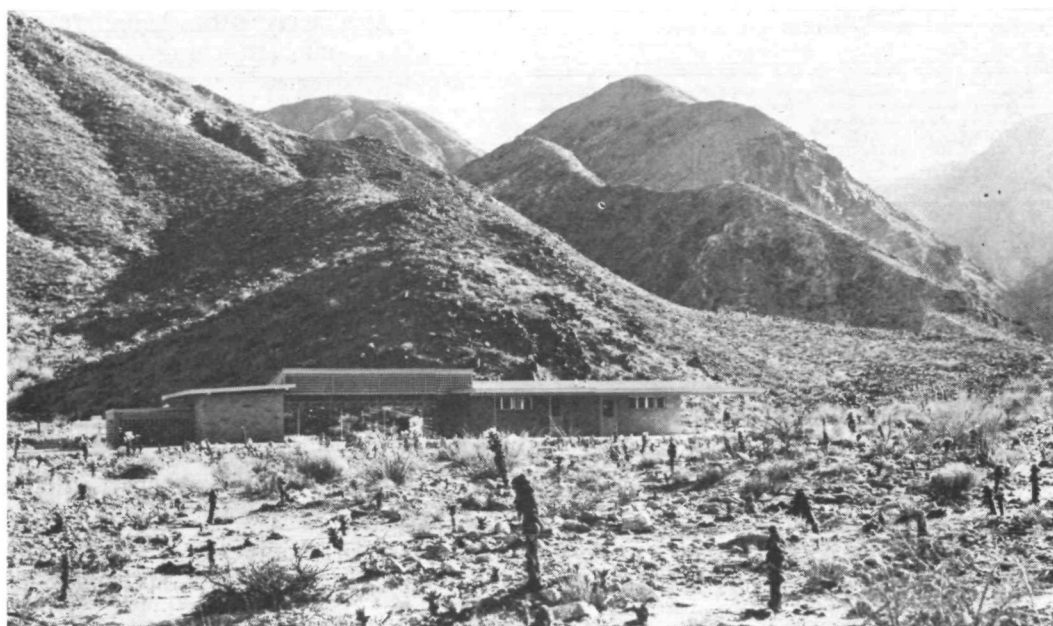
A view of the Philip L. Boyd Desert Research Center near the mouth of Deep Canyon, Riverside County, California. The air-conditioned laboratory and living quarters are on the right with the cistern and generators housed in the buildings on the left.
